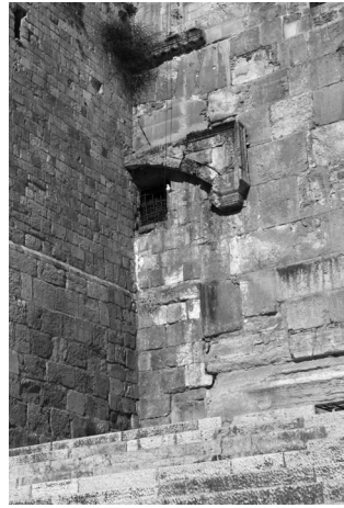
The remains of the Double Gates can be seen immediately above the protruding arch in the form of a half lintel and subtle arch. The wall made of small stones located to the left of the arch was constructed by the Crusaders in about AD 1099.
